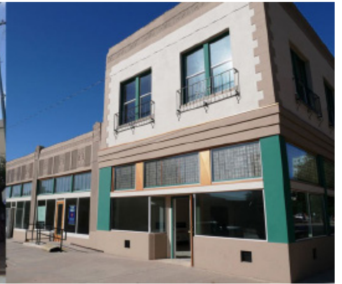
Post facade renovation
